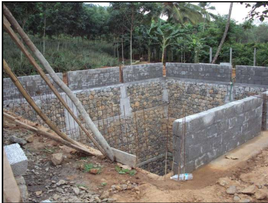
Photograph showing the construction of rain water harvesting tank
